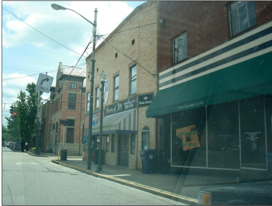
Figure 6. JOP 86, 312 Main St.
