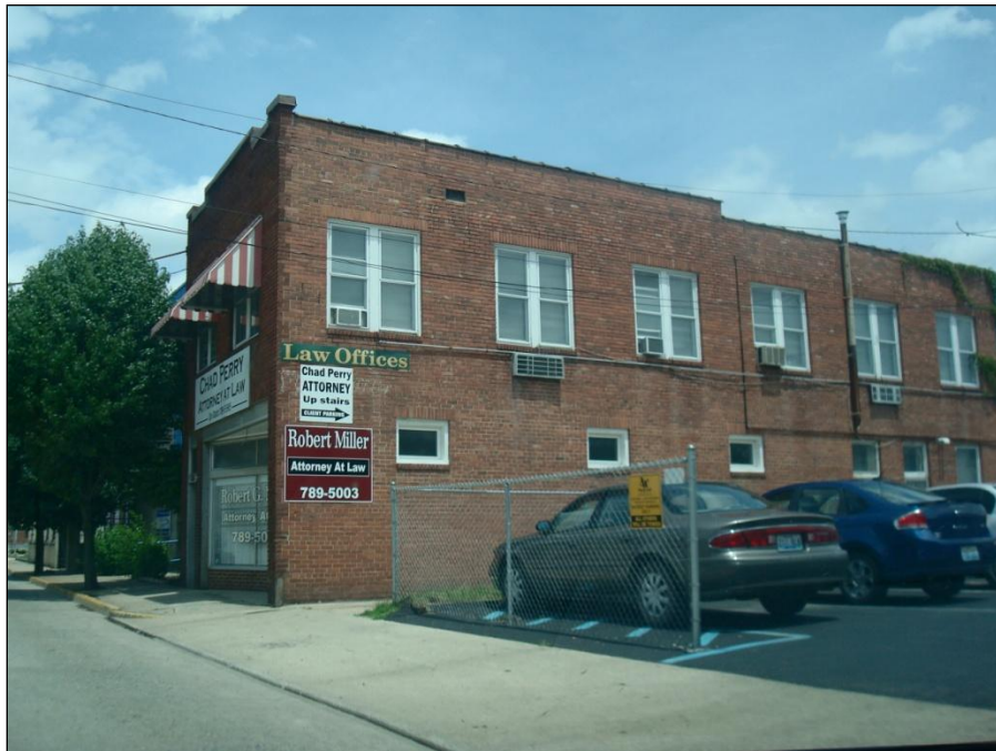
Figure 5. JOP 51, 216 Main St.
